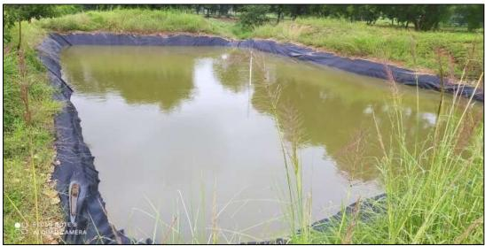
Fig 1. Farm Pond at full storage capacity
